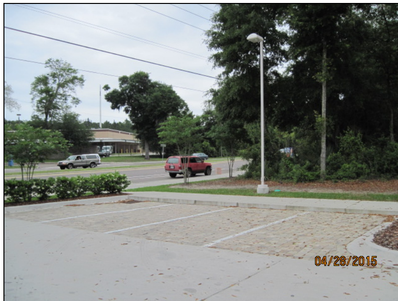
These four spaces will be removed to accommodate new right-out, exit only lane to McCormick Road.
